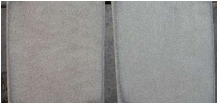
ZINCALUME® steel AZ150 Washed panels - Exposed for 21 years
