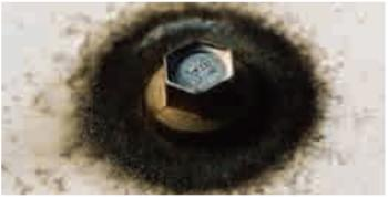
Fasteners used must be compatible with the selected cladding material. Stainless steel fasteners should not be used with galvanised ZINCALUME® steel or Clean COLORBOND<sup>™</sup> steel products.
