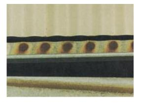
• Water flowing from a glass roof on to galvanized steel roofing (see photo below)
