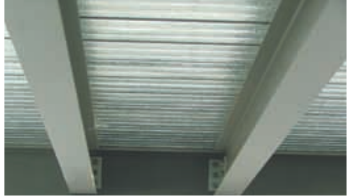
Galvanized steel decking
