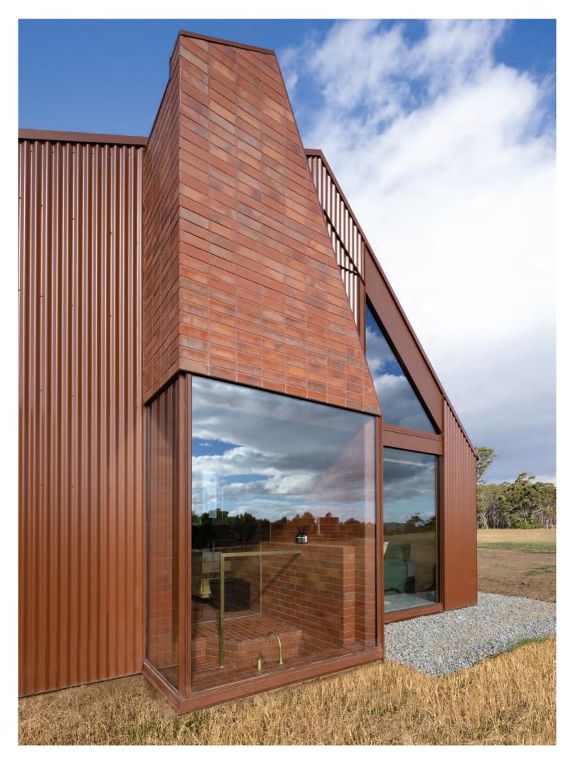
"We used COLORBOND<sup>®</sup> steel because it's lightweight, easy to transport, highly durable, easy to install and the colour is a strong reference and direct connection to the existing red-lead shacks on the island. It was always going to be steel"
