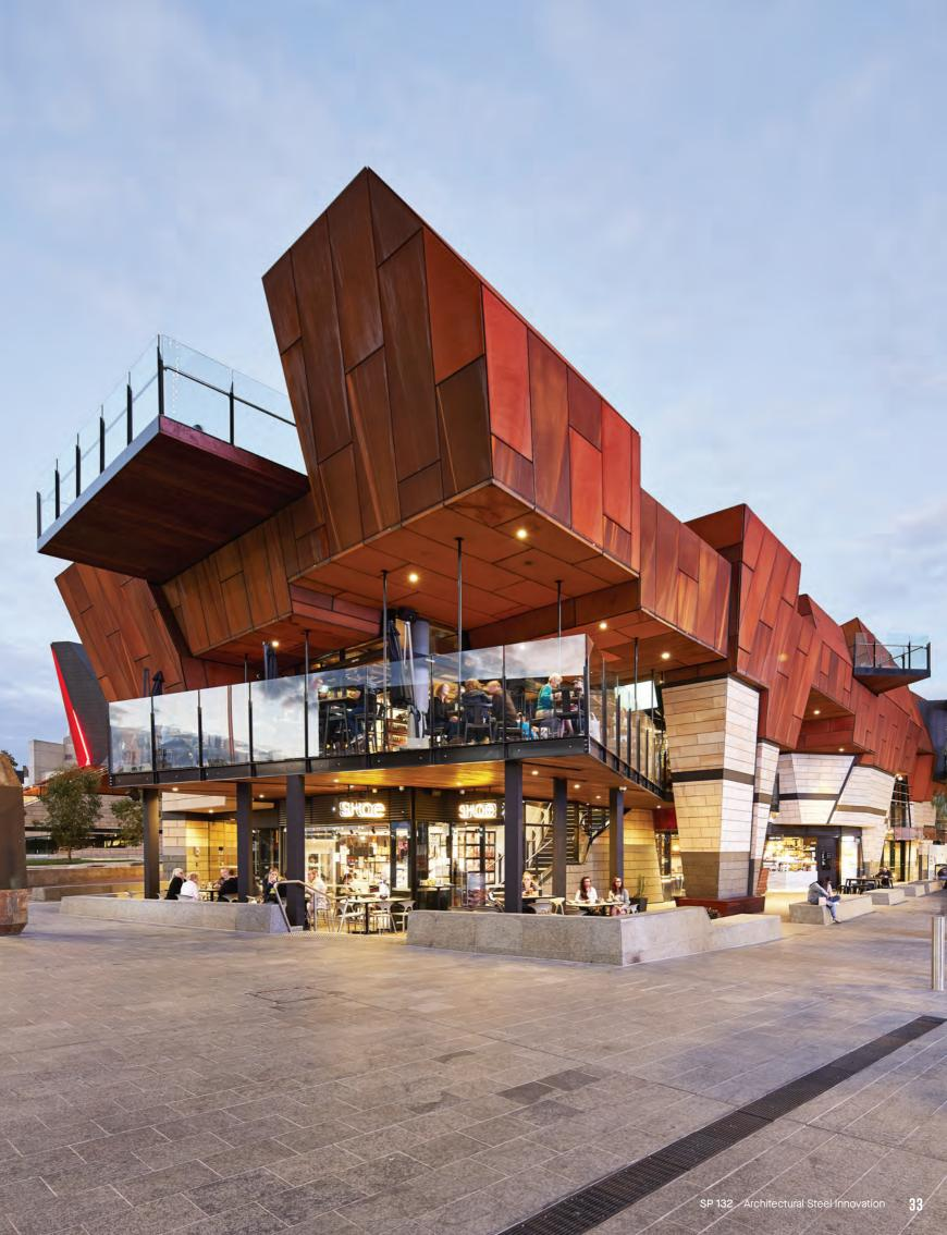
"Using steel that was sourced from local suppliers was vital to the overall design and its great strength-toweight ratio means we used less material to achieve more"
