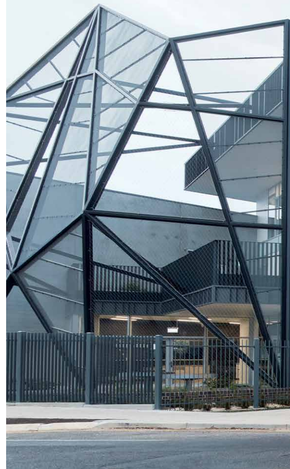
RIGHT: A footbridge comprising of steel, concrete, perforated aluminium screens, glass and CFC sheeting connects both sites together, allowing for simple, all-weather access between the existing building and the new development.
