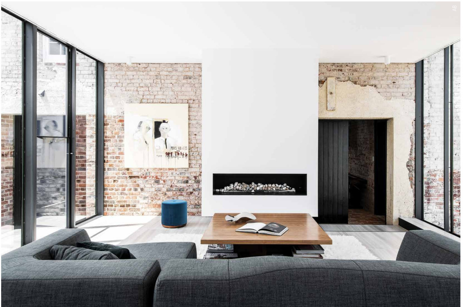
ABOVE: Inside the main living area in the new addition, spaces are kept open with custom fabricated slender steel mullions elegantly supporting the lightweight roof structure without the need for intrusive internal structural columns. BELOW: The rear wing of the existing Georgian building and its two symmetrical Georgian brick outbuildings have been connected and consolidated by a new lightweight glazed link custom framed with mullions fabricated from RHS.
