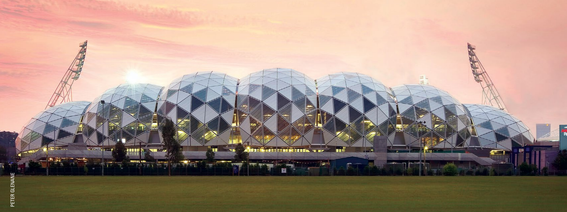
ABOVE: AAMI Park stadium, with its multi-faceted steel 'bioframe' design, is COX Architecture's stellar addition to Melbourne's world-class sporting precinct.
