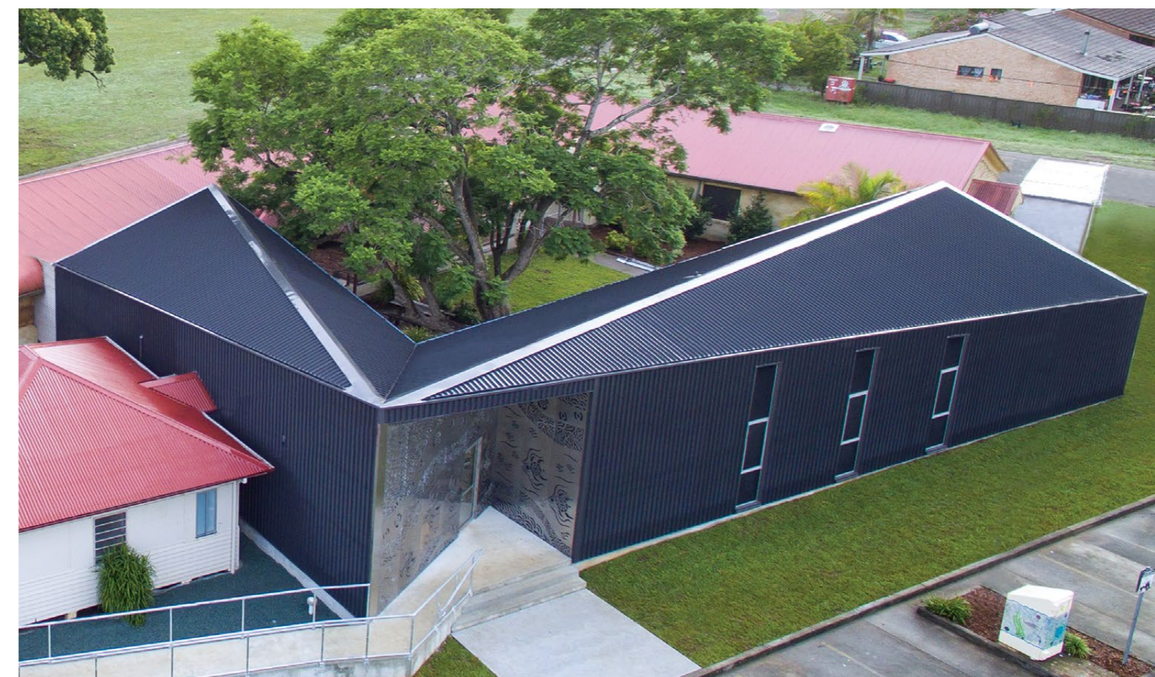
PROJECT Biripi Health Clinic CLIENT Biripi Aboriginal Corporation Medical Centre ARCHITECT Kaunitz Yeung Architecture PROJECT TEAM David Kaunitz, Ka Wai Yeung, Louis Wong STRUCTURAL ENGINEERING Bruce Hutchison, Chapman Hutchison ART SCREENS Vashti Gonda, Di Emme BUILDING SERVICES Lucid Consulting CIVIL Coast Plan PCA Boyce Consulting PRINCIPAL STEEL COMPONENTS Roofing and cladding made from COLORBOND® steel in LYSAGHT LONGLINE 305® profile, in the colour Monument® PROJECT TIMEFRAME Commenced May 2016, completed March 2017 AWARDS 2018 Australian Institute of Architects New South Wales Chapter Awards: COLORBOND® Award for Steel Architecture; Premier’s Prize for distinguished social merit; Commercial Building Award. 2017 European Healthcare Design Award: Healthcare Design Award, and Infill or Conversion Award. 2017 World Architecture News Awards: Finalist, Healthcare BUILDING SIZE GFA: 275m² TOTAL PROJECT COST $1 million, including GST
