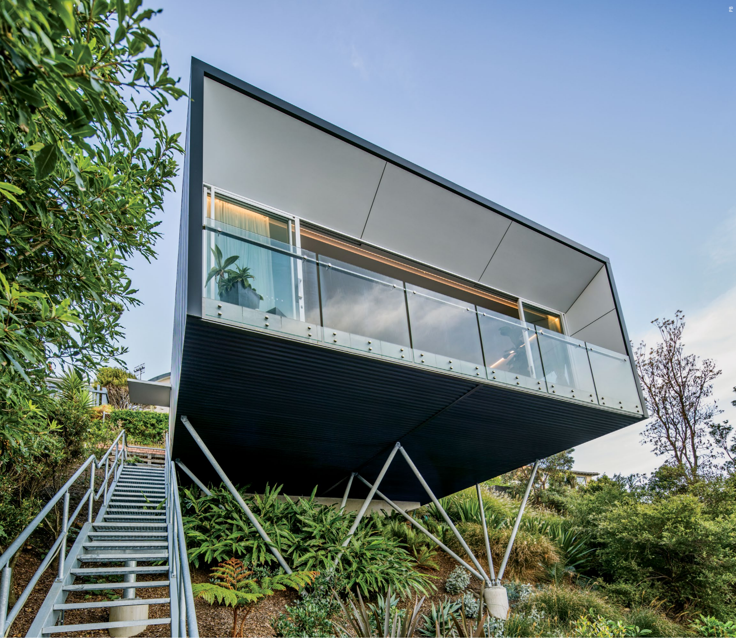
ABOVE: The wall cladding made from COLORBOND® Ultra steel in LYSAGHT SPANDEK® profile, in the colour Monument®, wraps under the studio's soffit. RIGHT: The CHS piloti also provide cross-bracing for the overall structure, resulting in a clean aesthetic.
