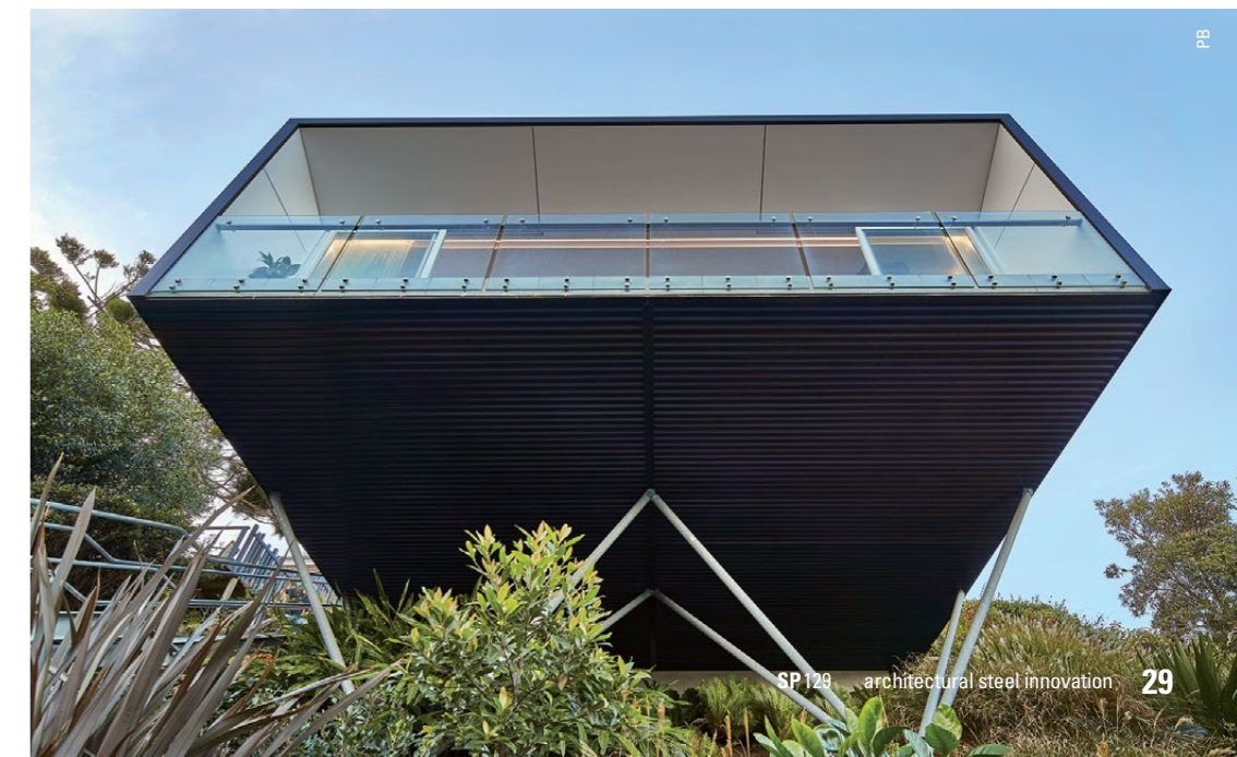
ABOVE: The wall cladding made from COLORBOND® Ultra steel in LYSAGHT SPANDEK® profile, in the colour Monument®, wraps under the studio's soffit. RIGHT: The CHS piloti also provide cross-bracing for the overall structure, resulting in a clean aesthetic.
