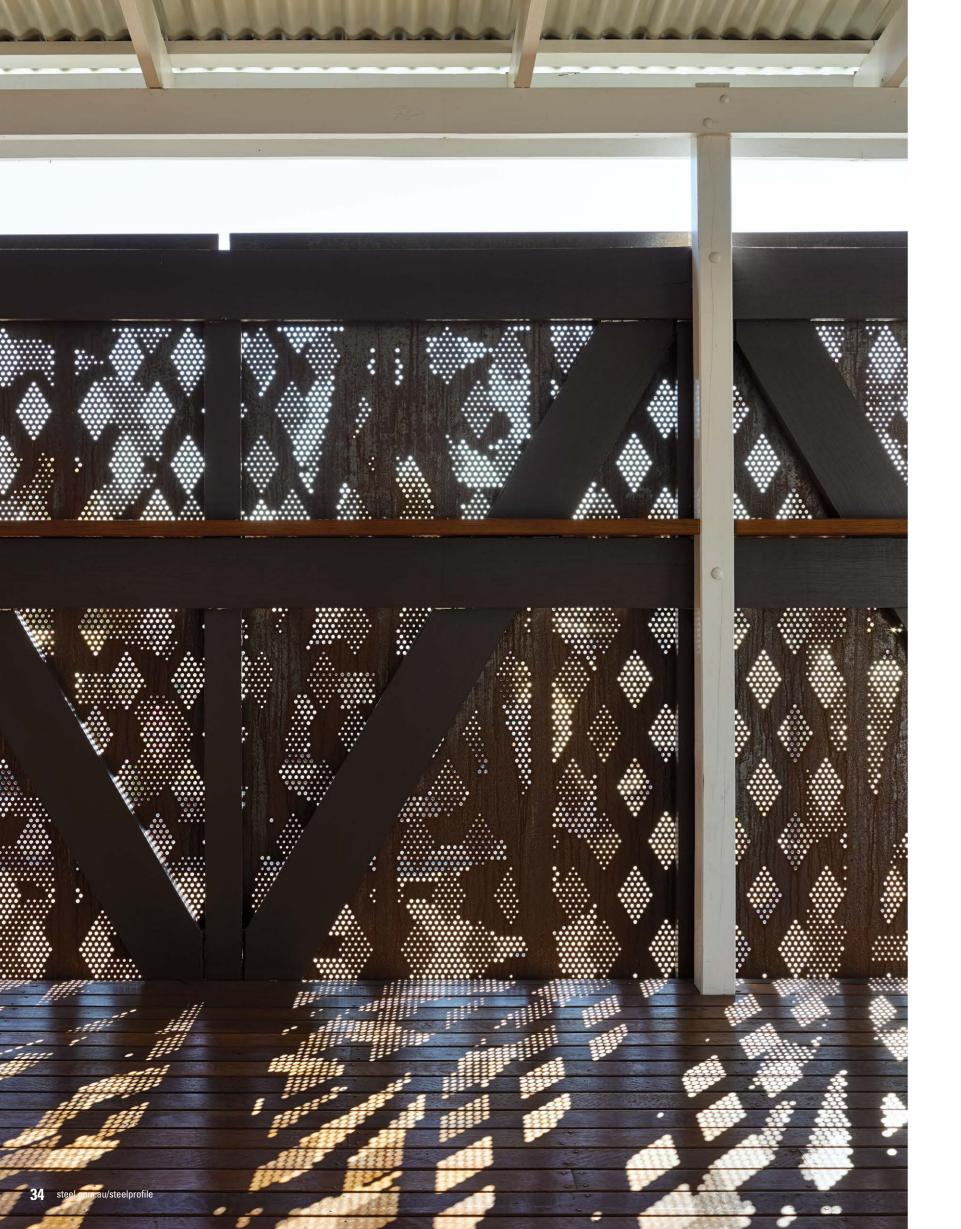
OPPOSSITE: The panels made from REDCOR® weathering steel create a winning shadeventilation combination for the harsh outback environment.
