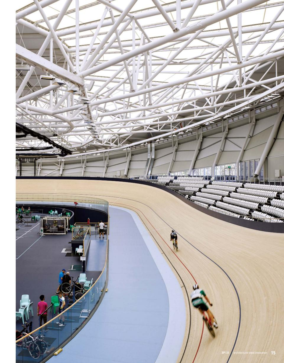
"We chose to use fillet-welded saddle plates on site rather than bolted splices. This meant that major elements of the roof structure could be lifted in, positioned on welded saddle connections and fillet-welded, providing flexibility in terms of tolerances.
