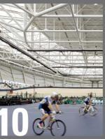
Cox Architecture's design for Queensland's first enclosed cycling track employs 1200 tonnes of steel in an efficient engineering solution for its vast and graceful, saddle-shaped roof structure.
