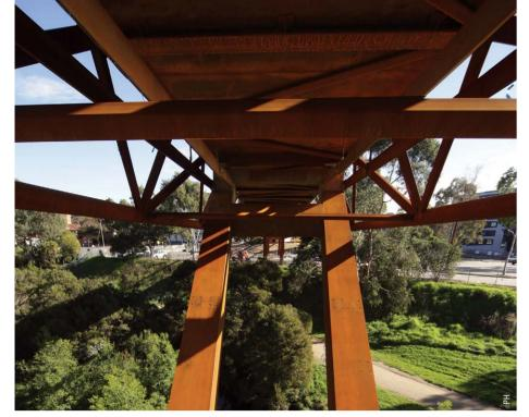
ABOVE: The underside of the bridge resembles a seamlessly integrated structure and platform, thanks to the 'baking trays' -- made from 3mm-thick REDCOR® steel coil in 1594 HW350 grade -- that provide permanent formwork for the concrete deck.
