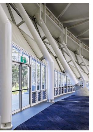
ABOVE: Nine-hundred tonnes of circular hollow sections and 300 tonnes of steel plate, including custom-welded tapering pin joints made from XLERPLATE<sup>®</sup> steel, were fundamental in achieving the twisting shapes of the saddle-like roof.
