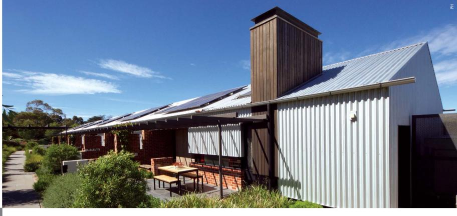
ABOVE AND BELOW: The northern elevation features cladding made from ZINCALUME<sup>®</sup> steel in LYSAGHT CUSTOM ORB ACCENT<sup>®</sup> 35 profile as a mediating screen for individual suites, offering privacy and solar control. A simple pergola will eventually be vine-covered to provide dappled shade. The rippled steel surface produces a sun dial effect of moveable shadow and light.
