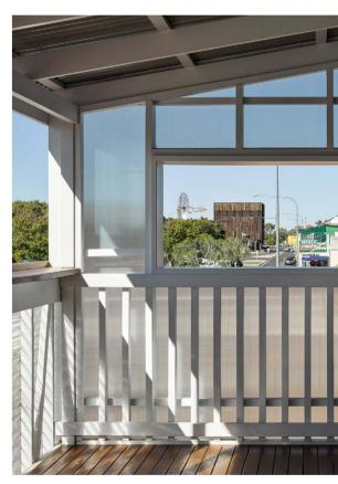
LEFT: Roofing and guttering made from COLORBOND® steel in the colour  $\mathsf{Surfmist}^{\scriptscriptstyle{(\!\!\!\!\)}}$  was designed and fabricated to integrate neatly with the flashings and polycarbonate screens.
